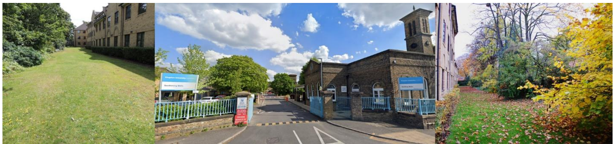
Figure 3.8.a: Photos of Seething Wells halls of residence
