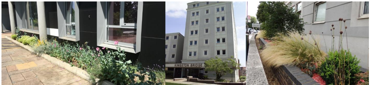
Figure 3.9.a: Photos of Kingston Bridge House
